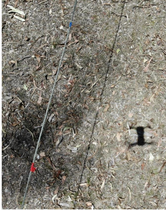
Figure 12 Red and blue markings on the conductor surface
