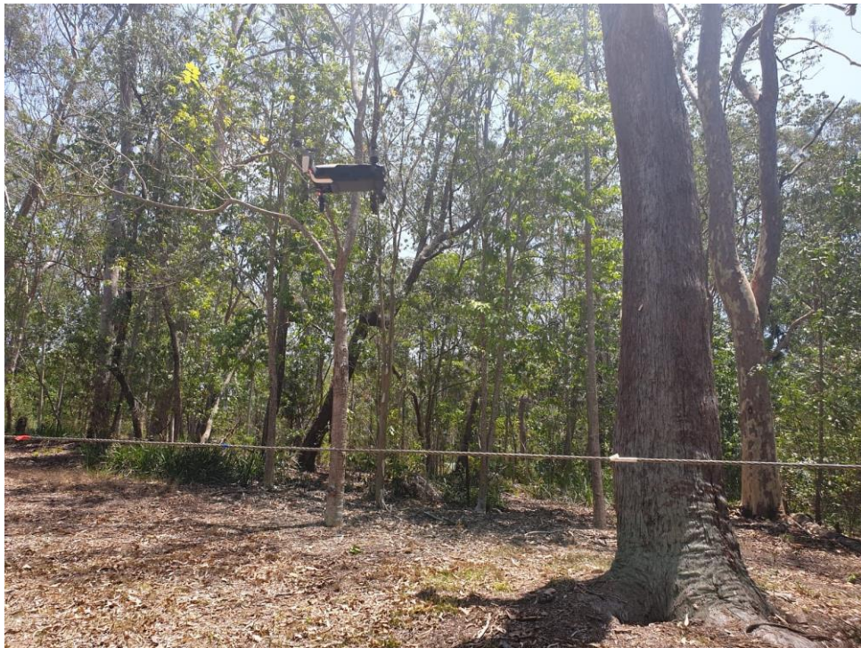
Figure 7 Conducting drone based visual inspections of a copper conductor in an outdoor location
