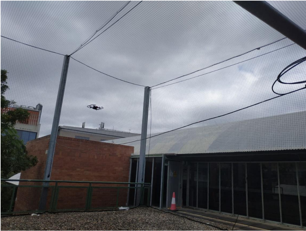
Figure 8 Conducting drone based visual inspections of a copper conductor in a dedicated drone flying zone
