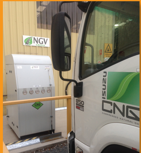
A Gouge Linen CNG Isuzu with their on-site CNG refuelling compressor.
