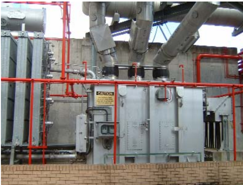
Figure A1. Cabling between large transformer and switchboards
