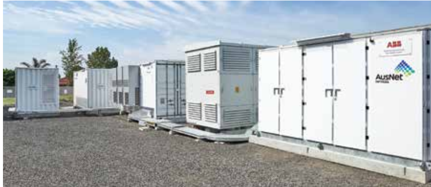
Grid Energy Storage System Installation
