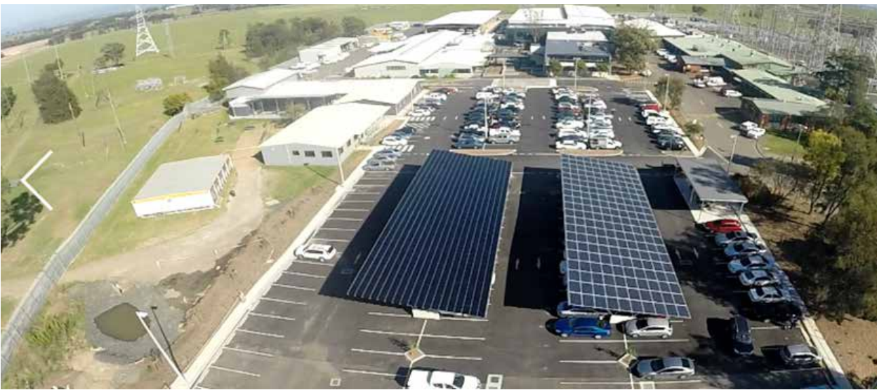
FIGURE 2 WALLGROVE SITE WITH THE 98.4 KW OF SOLAR PANELS
