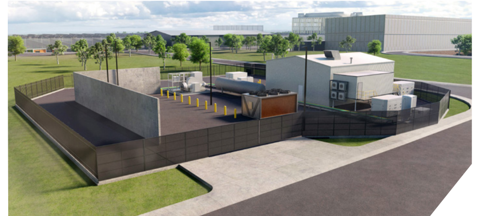
AGIG's Hydrogen Park in Tonsley Innovation District in SA
