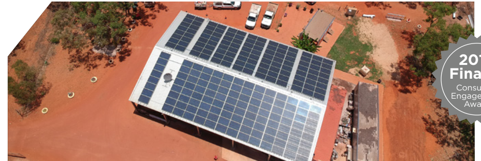
Horizon Power's solar installation at the Djarindjin roadhouse in the Kimberley, WA
